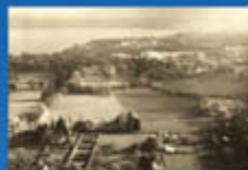
The building site 1959
