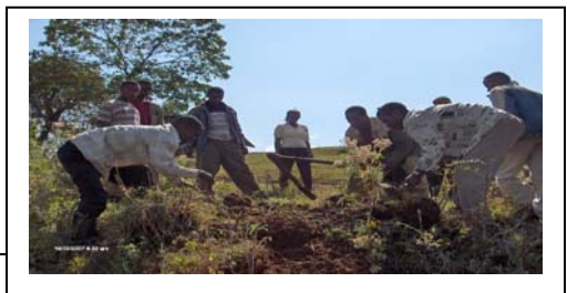
Construction of community latrines in Gooroo district (17/01/07)
