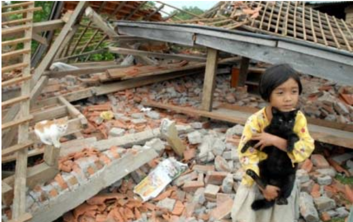
Caption: Disaster victim and damaged house in Jambi
