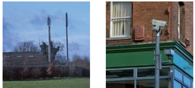
Figure 4.1 Photos of mobile phone mast and microcell-antennas.
