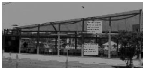
Fig. 1 The “outdoor” addition to a club in New South Wales, Australia where the law currently allows smoking in this type of outdoor area. (Photo courtesy of ASH Australia)
