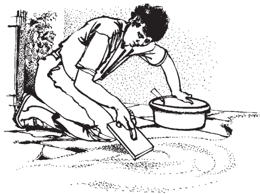
Fig. 3.19 Resting places in floors can be filled and covered with a layer of cement.
