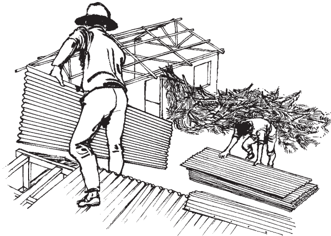
Fig. 3.21 Corrugated iron sheets do not offer a suitable habitat to triatomine bugs.
